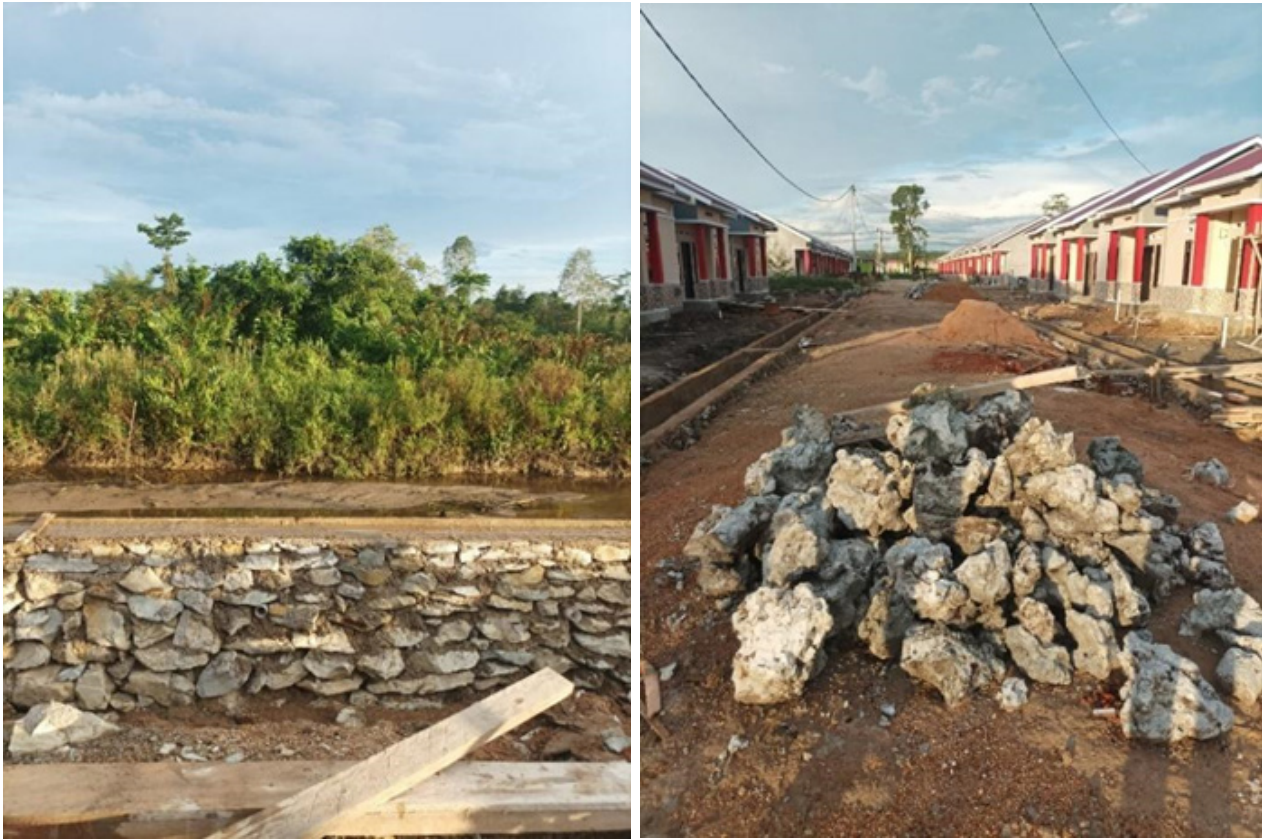
Picture 1 Building Riprap and Settlement Made of Coral Reefs, Sands, and Gravels
